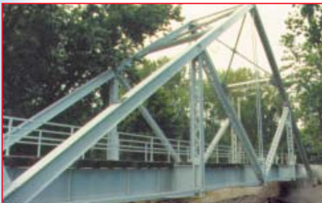
Under a Section 106 agreement, the U.S. Army Corps of Engineers dismantled and stored one of the Nation's last historic Waddell A-Truss bridges to save it from flood damage during construction of Smithville Lake in Missouri. Collaborative efforts led to its reconstruction in a local riverside park.
